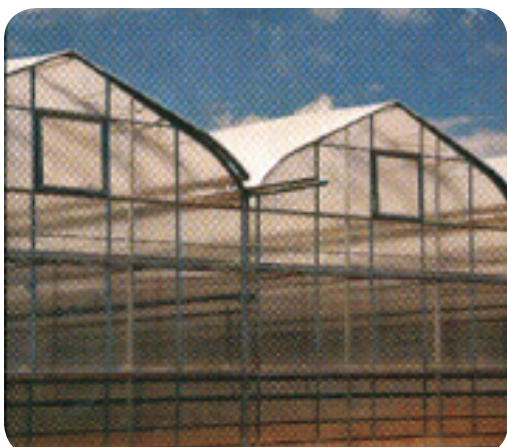
(Above) A gutter-connect greenhouse covered in Lexan Twinwall Polycarbonate.
